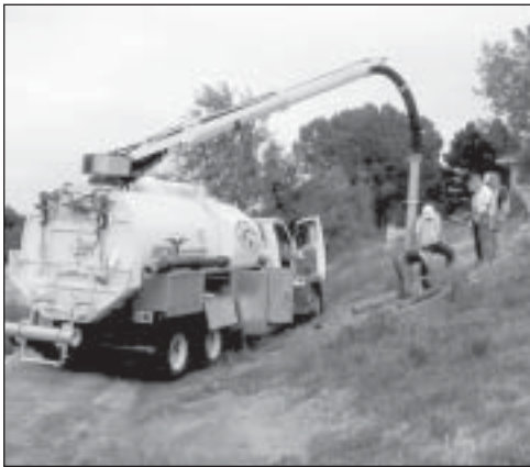
Water Shutoff Repair
