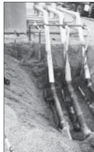
Live Gas Lines Exposed
