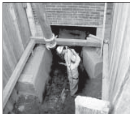
Repairing Steam Line Under Foundation
