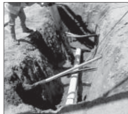
Live Gas Lines Exposed
