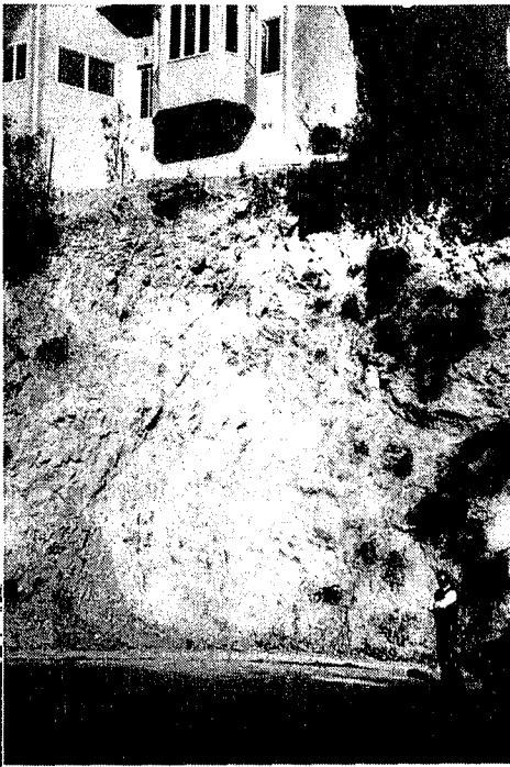
FIG 1 MULTI-MILLION DOLLAR HOME ON FAILING CLIFF FACE OVERLOOKING THE PACIFIC OCEAN BEFORE SLOPE STABILIZATION USING WATER JET TECHNOLOGY
