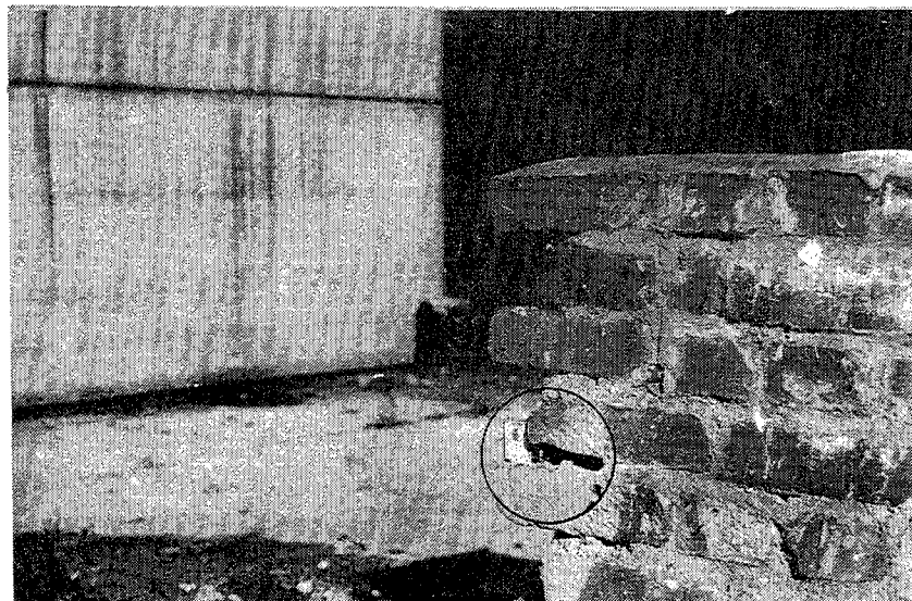
Fig.5. THE SLOT WAS CUTTING BY WATER-SAND JET
