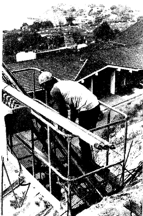
FIG 5 MAN LIFT PLATFORM WITH WATER JET DRILL ON FACE
