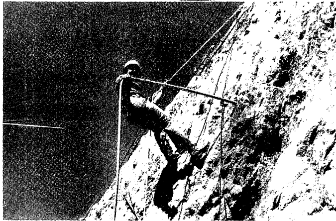
FIG 11 DRILL CUTTING AND WATER BEING REMOVED FROM TIEBACK HOLE WITH COMPRESSED AIR
