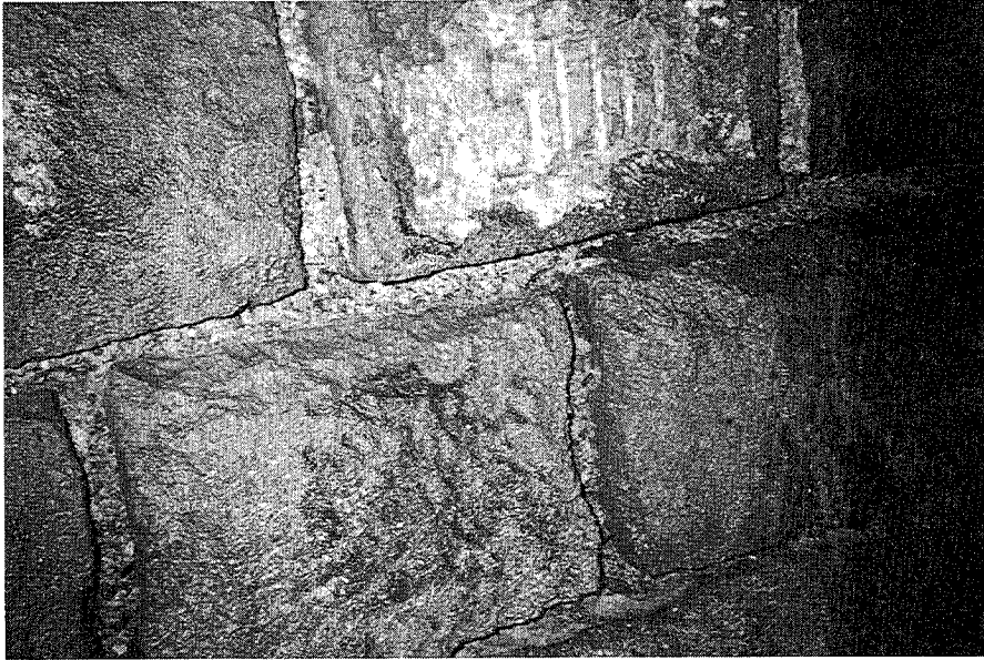
Figure 4. Tunnel wall after cleaning and removing of joints filling
