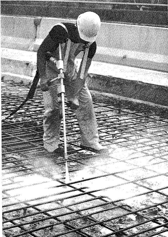
DESCALING OF REBAR AT 10,000 PSI
