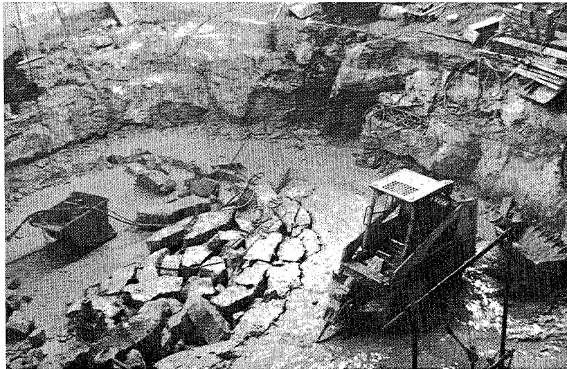
Figure 7. Pattern of blocks broken out in the floor of the excavation.
