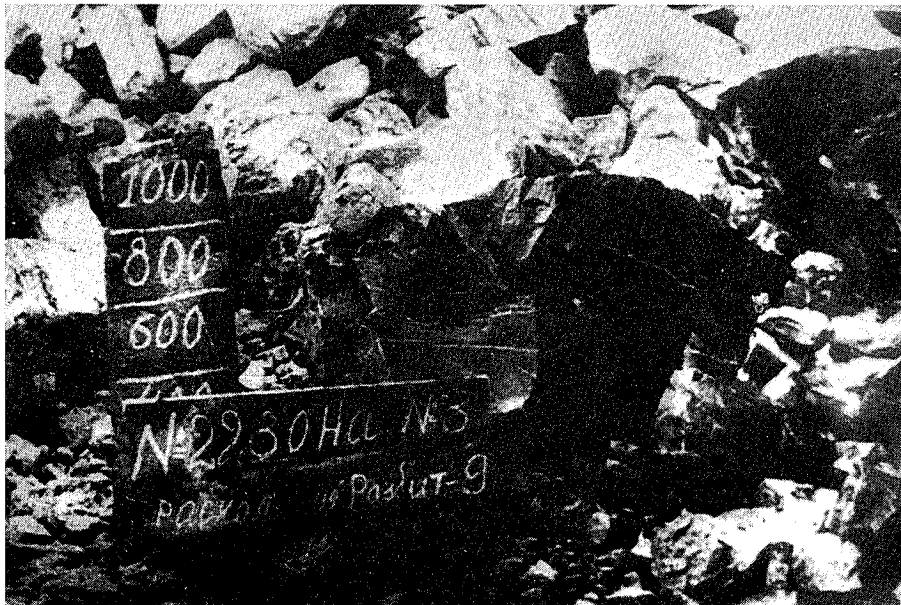
Figure 5b Breaking of the sandstone lump – after 9 shots.
