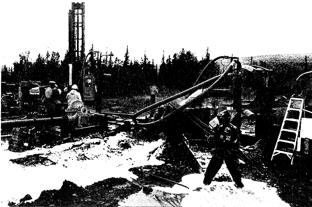
Figure 11. Borehole mining at Tenderfoot Creek, Alaska.
