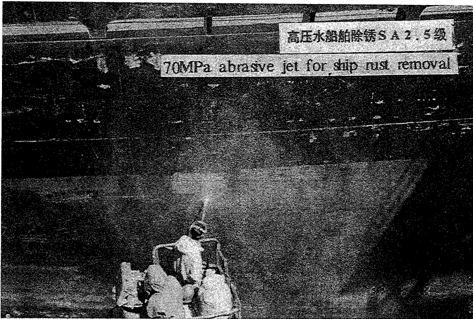
Fig.8 Worksite of shiphull rust removal
