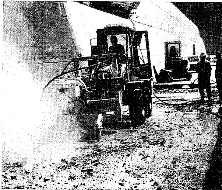
Figure 1. Concrete Hydrodemolition Unit. (Photo: WOMA GmbH, Duisburg)
