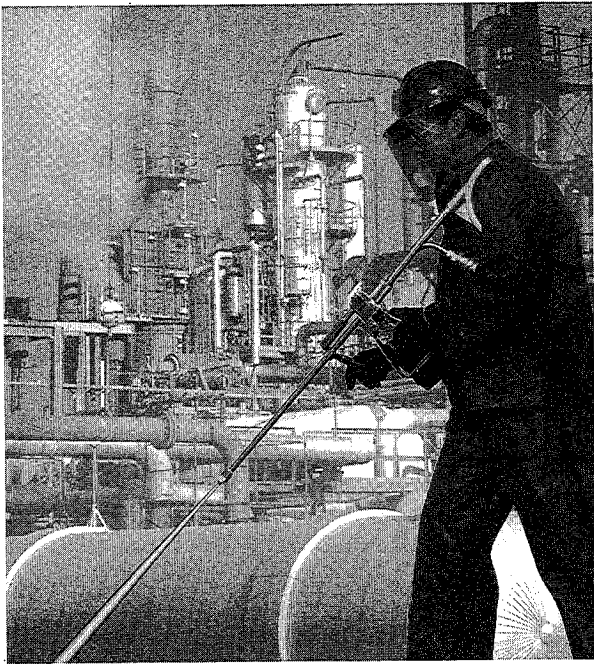
Figure 1. Water jetting is the most common cleaning method used in the petrochemical industry.
