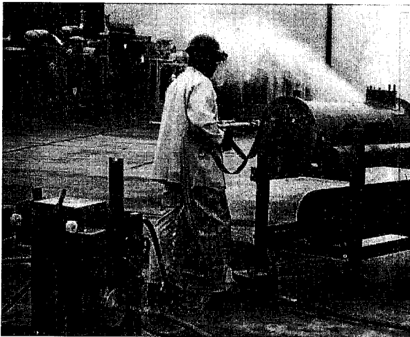
Figure 7. Small semi-automated flex lance machines take the lance out of the operator's hands.
