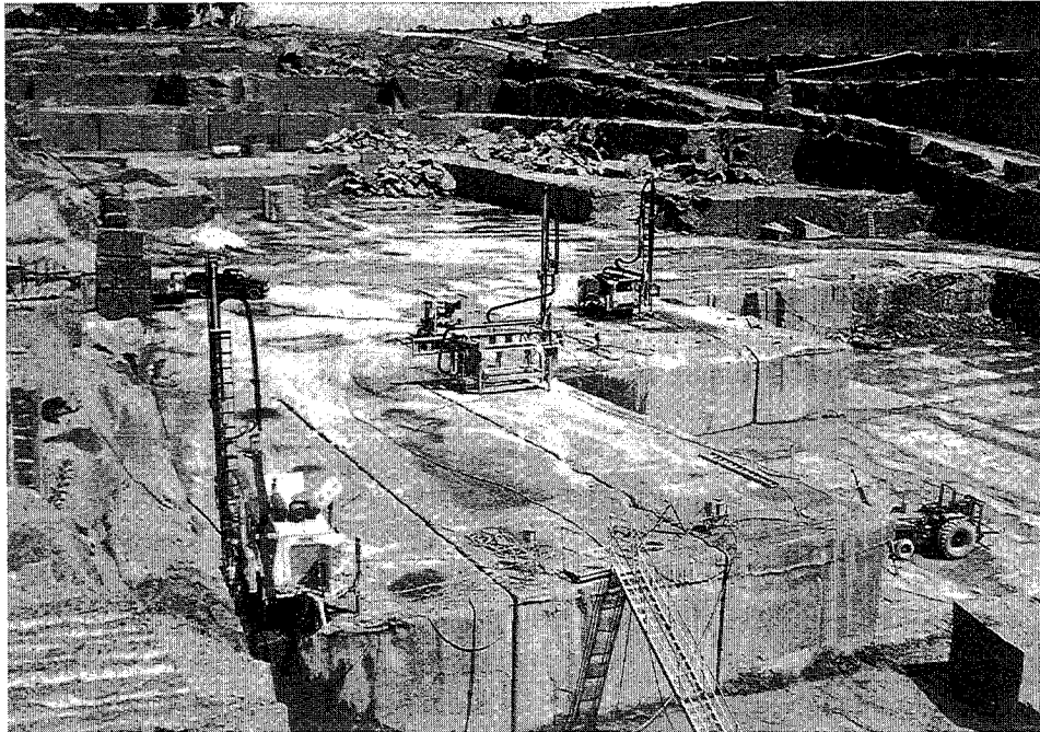
Photo #2 — Bench Gantry
